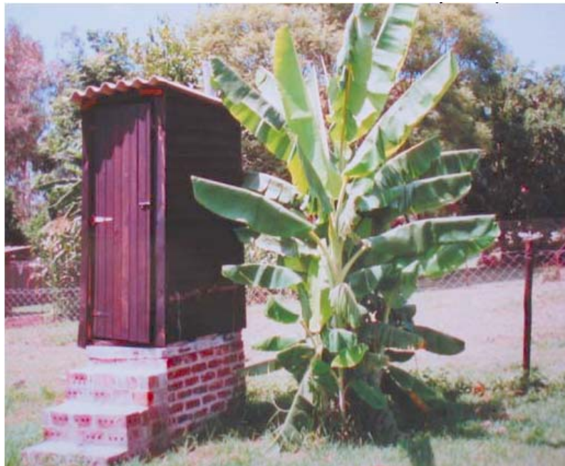
Figure 1: Banana growing on a soil composting toilet after its period of usage. The structure presented beside alternates as an Arborloo and Fossa alterna . (Morgan, 2004)
